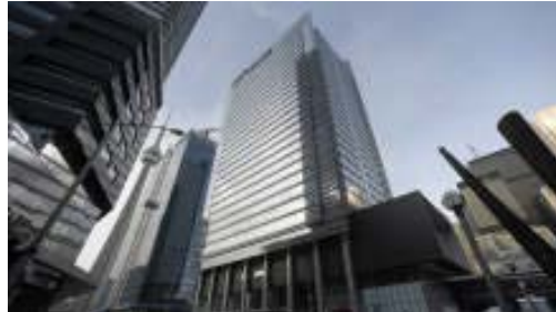
The new Telus Tower in downtown Toronto is a showpiece of environmental design and energy efficiency, one of the traits in a workplace sought by younger workers.
